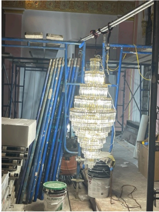
Completion of the Balcony Renovation
