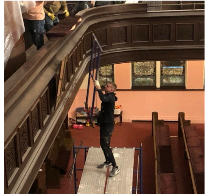
Completion of the Balcony Renovation
